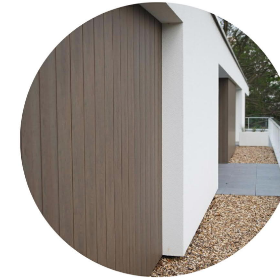
VERTICAL PANEL SIDING: TRESPA - PURA - HIGH PRESSURE LAMINATE PANEL - FINISH: AGED ASH
