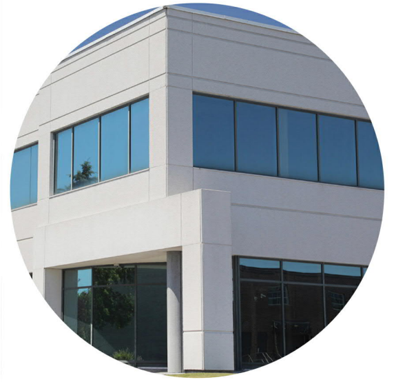
EIFS: DRYVIT - EIFS - FINISH: REPOSE GRAY
