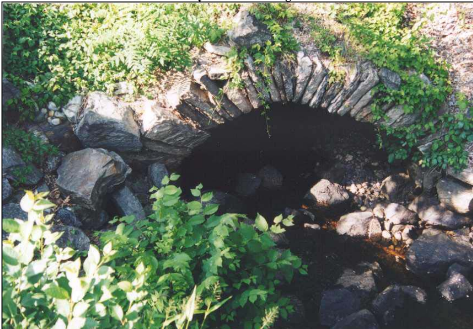
Keystone Arch Bridge
